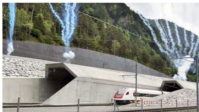
The first train emerges from the tunnel
